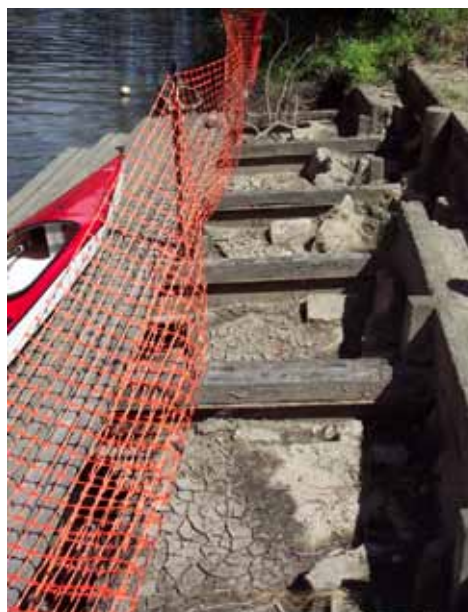
FCC landing under repair.
